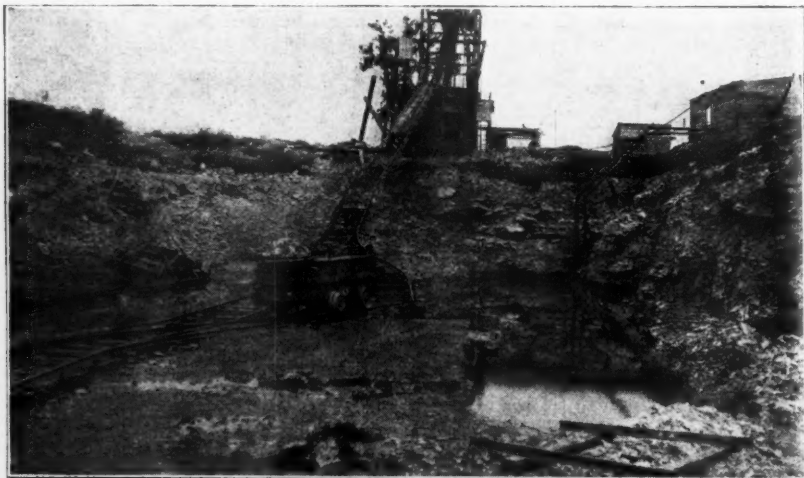
Cars Carry Blasted Rock to Crusher
